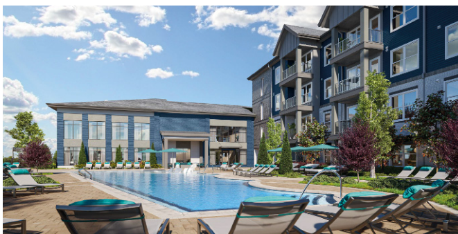
BVT Residential USA 17, Referenzobjekt „Aventon Gwynn (Exchange)“ nahe Atlanta, Georgia
